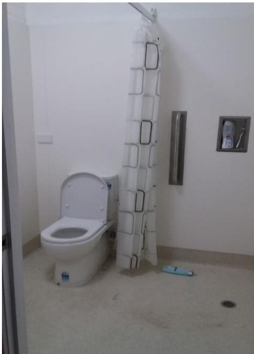
Anti-ligature bathroom (withdrawal unit)
